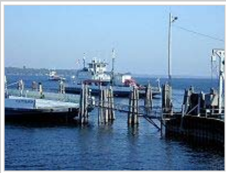
The LCTC ferry slip at Grand Isle, Vermont.
