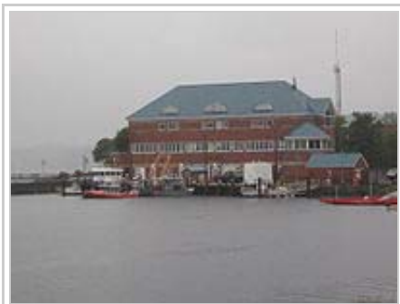
USCG, Burlington, Vermont - main installation.
