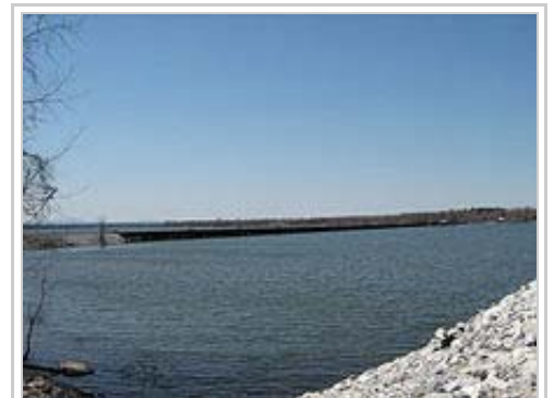
The Swanton-Alburgh trestle spans Lake Champlain between the two Vermont towns, a distance of about .8 miles (1.3 km)
