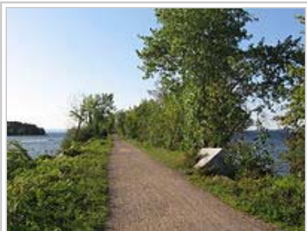
The causeway connecting Colchester and South Hero.
