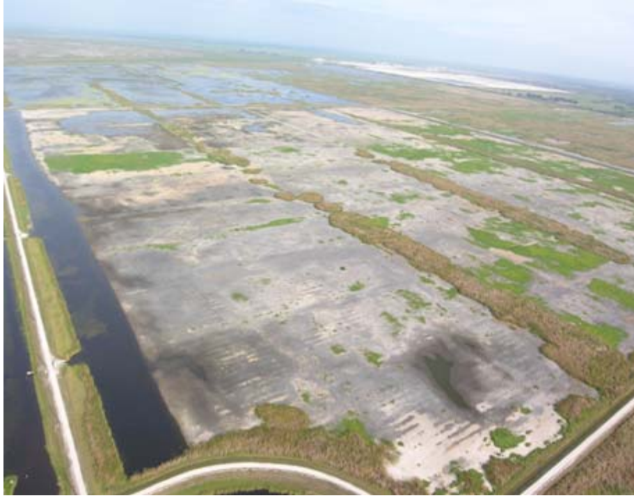
Figure 5-19. An aerial photo of STA-1E, Cell 4, in May 2009, showing cell dryout, resulting in loss of SAV (photo by the SFWMD).
