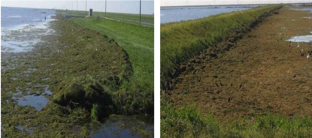
Figure 5-80: Photographs of SAV "roll-up" in (A) STA-2, Cell 3, and (B) STA-1W, Cell 5B, following Hurricane Wilma in 2005 (photos by the SFWMD).
