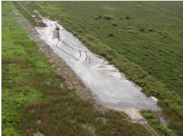
308 Figure 5-8. Location of degraded berm in STA-1E Cell 2 at the former Periphyton 309 STA Demonstration Project site (a), and photo of the degraded berm (b) (photo by 310 the SFWMD). Approximately 500 linear feet of the berm was degraded as an interim 311 measure to allow for more flow through the Eastern Flow-way of STA-1E.
