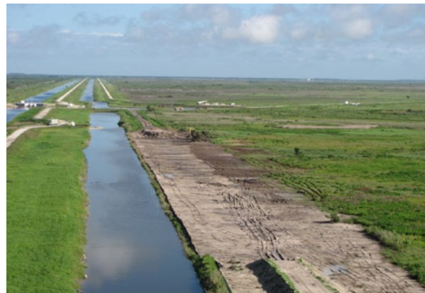
Figure 5-38. A portion of a redundant levee in STA-6 between the G-601 and G-602 structures (top photo); approximately 2,800 linear feet of levee was removed (bottom photo) and the spoil material was used in Cell 5A for the environmentally sensitive area protection (photos by the SFWMD).
