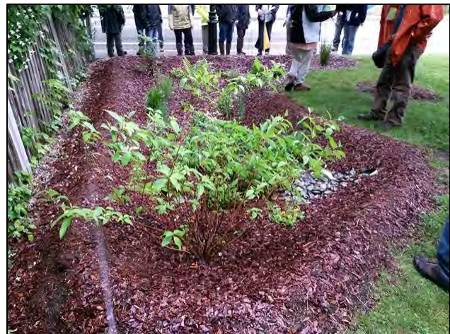
Rain gardens are an excellent way to retain and infiltrate stormwater on most residential sites.
