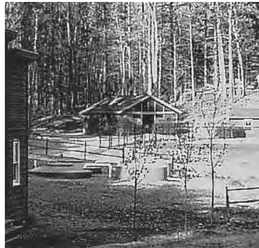
Camp Thoreau – the round treatment tanks (center area) are located amongst the camp buildings and next to the recreation fields. The buildings are for camp activities.
