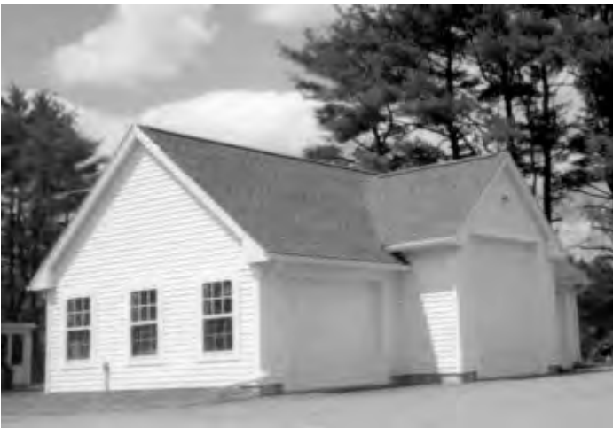
A large building for an above ground cluster system
